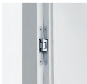
Door frame corner from hinges side
